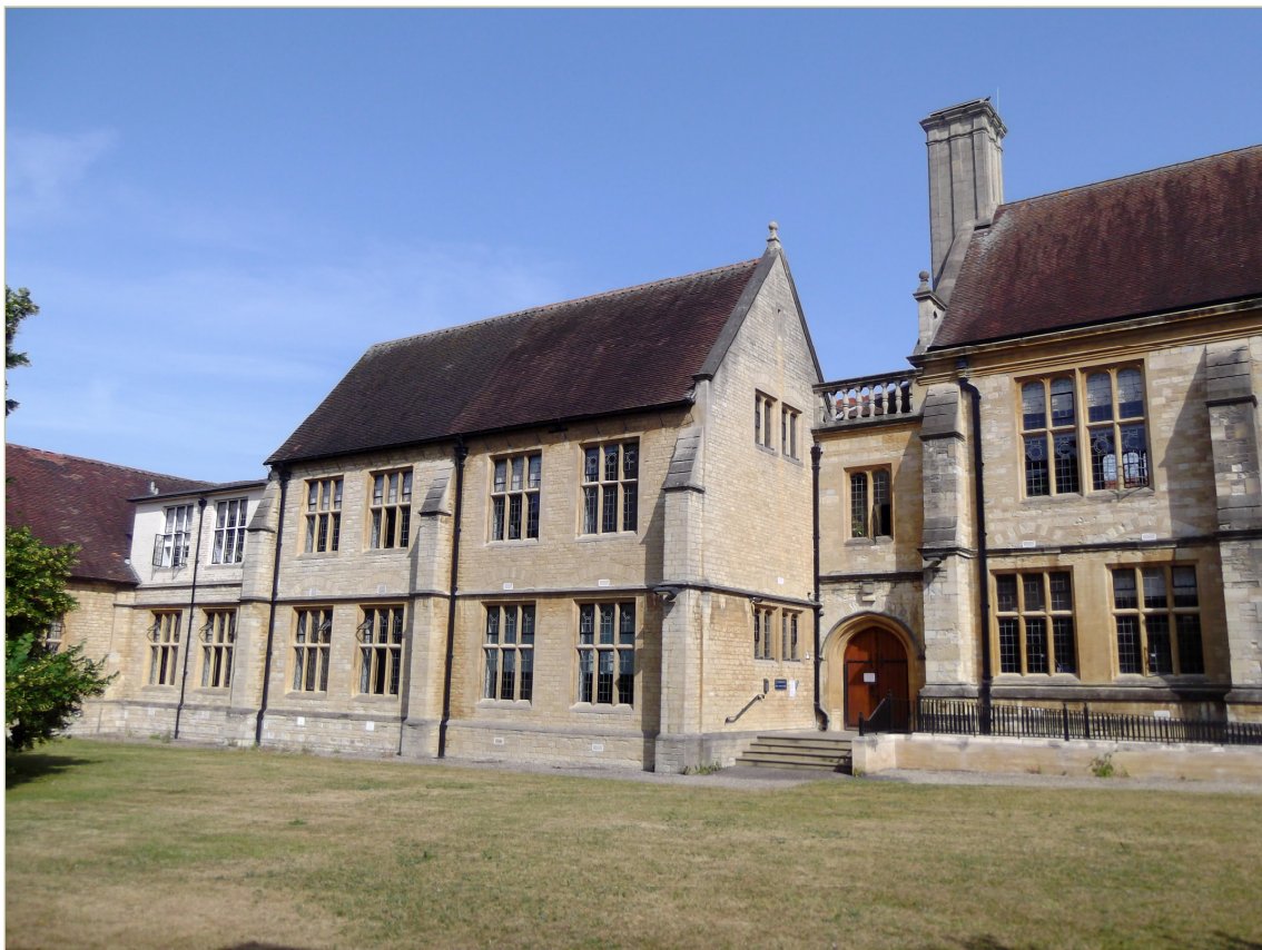
Figure 14. The rear elevation looking north-westwards. The original Jackson building, which includes the entrance, is on the right of the image. The first bay immediately to the left of the entrance is Jackson’s 1892-5 extension. The next bay onwards represents the 1915 extension, apart from the flat-roofed first-floor section, which probably dates from 1935.
