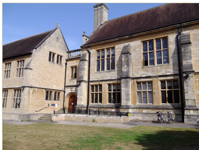
Figure 18. Ramped access to the main, rear entrance
