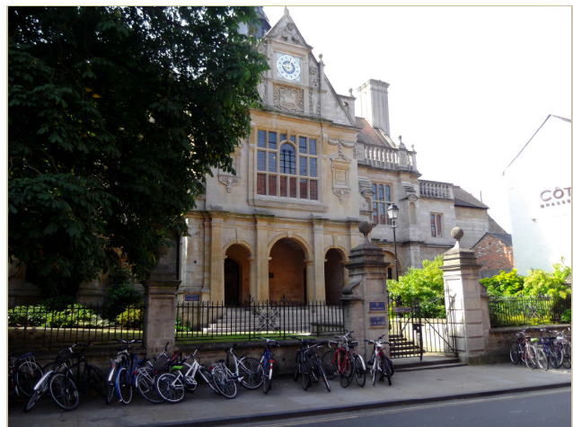
Figure 11. 11.1, top, the piers and screen approached from the west. 11.2, centre, the northern elevation revealed behind the screening buildings. 11.3, bottom, the northern elevation from across the street
