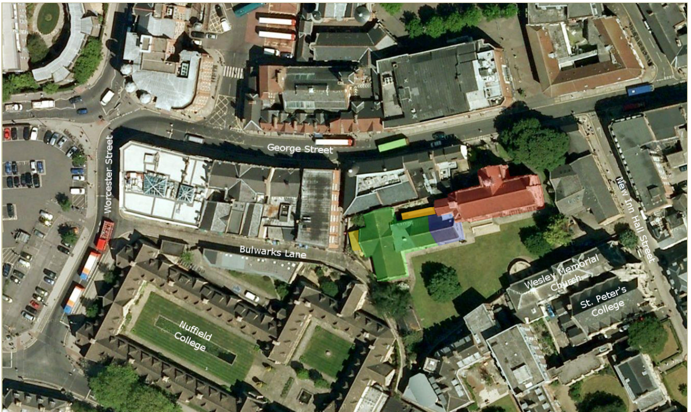
Figure 1. Satellite image of the Old Boys' High School and the surrounding area. The original 1880-1 Jackson building is highlighted in red. His 1892-5 extension is highlighted in blue. The 1915 extension is highlighted in green. The 1935 extension is highlighted in yellow and the 1977-8 toilet extension is highlighted in orange
