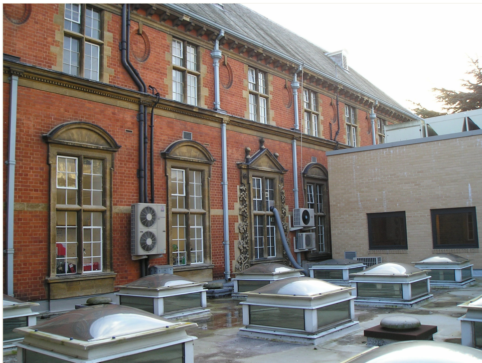
Figure 3. Photograph of northern elevation, January 2007. The ground floor is obscured by later additions. The embellished central window from Figure 2 can be identified third from the left.
