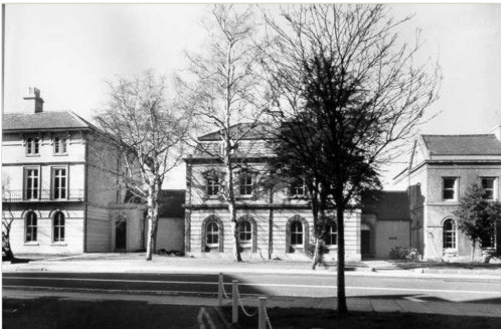
Figure 3. 9 to 15 Banbury Road in the late 1970s, showing newly-constructed connecting corridors.
