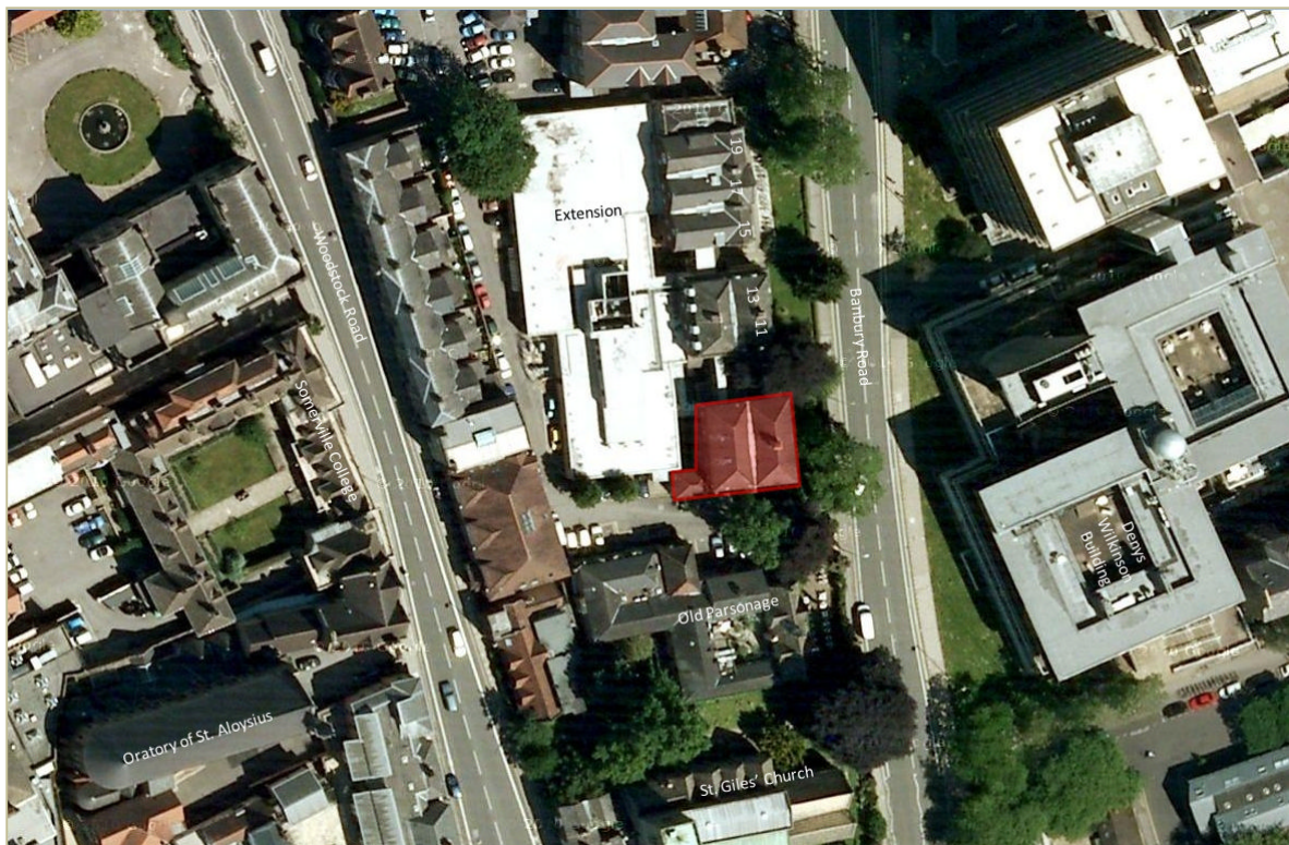
Figure 1. Satellite image of 7 and 9 Banbury Road (outlined in red) and the surrounding area, orientated with north at the top of the image
