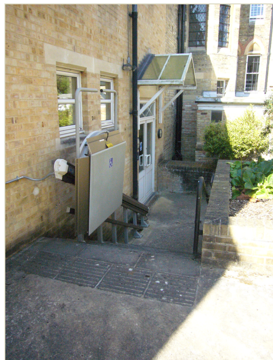
Figure 5. Disabled access at the rear of the building
