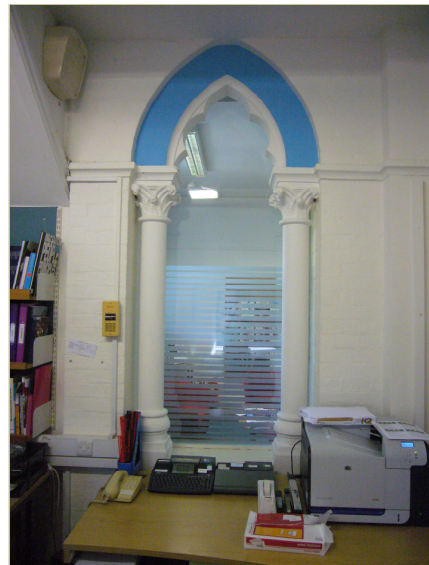
Figure 10. Top Left, cornice moulding and iron pipe brackets. Top Right, external windows converted to an internal archway. Bottom Left, Moore's conservatory, the ceiling obscuring Georgian wired glass. Bottom Right, external window converted into internal window
