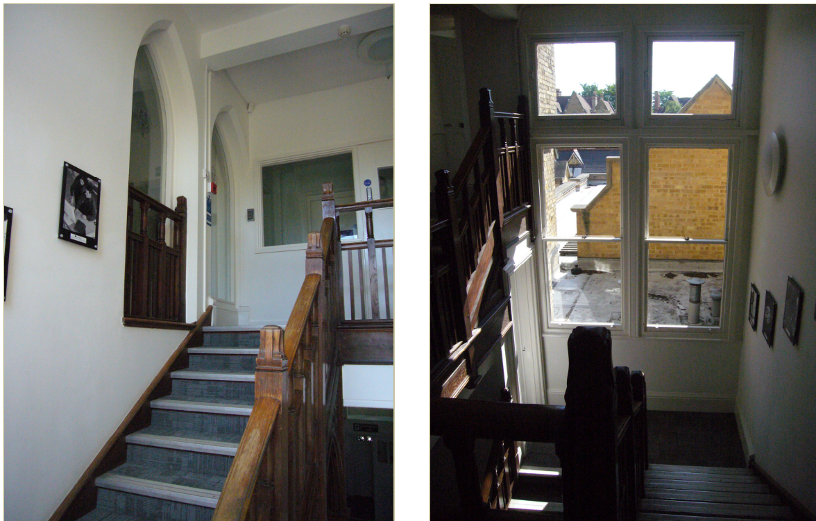
Figure 9. Left, the first-floor landing looking west. Right, the rear window looking east
