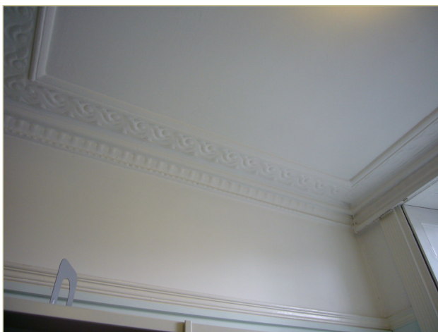
Figure 16. Top left, the utilitarian character of the first-floor common room. Bottom left, ceiling decoration in the ground-floor front room. Right, joinery on the staircase
