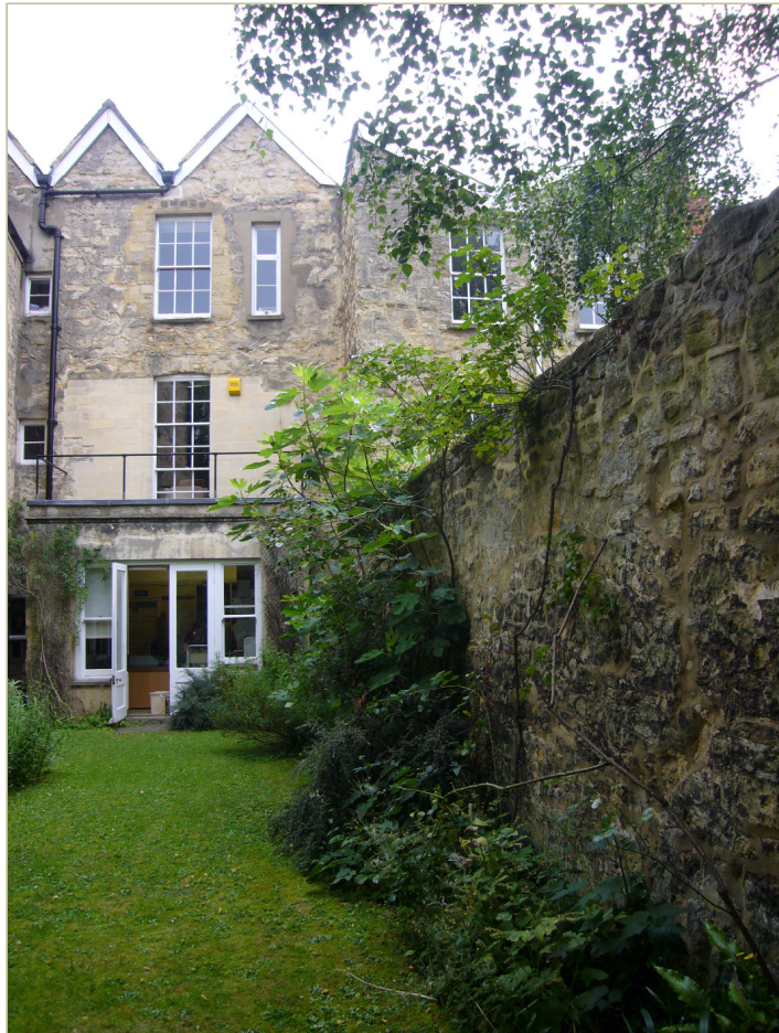
Figure 11. The rear elevation and garden wall
