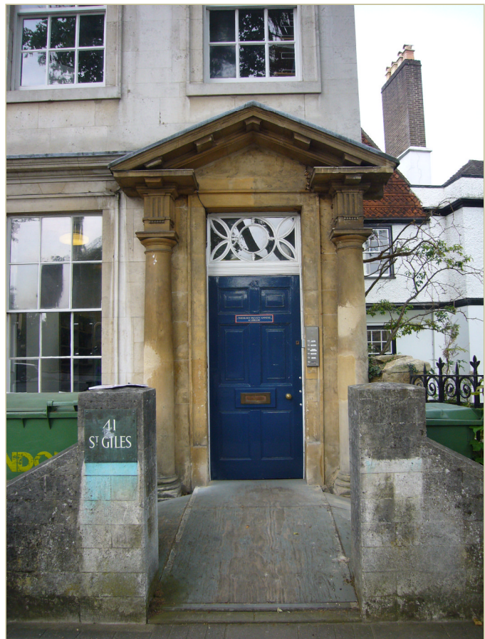
Figure 15. The main entrance from St. Giles'
