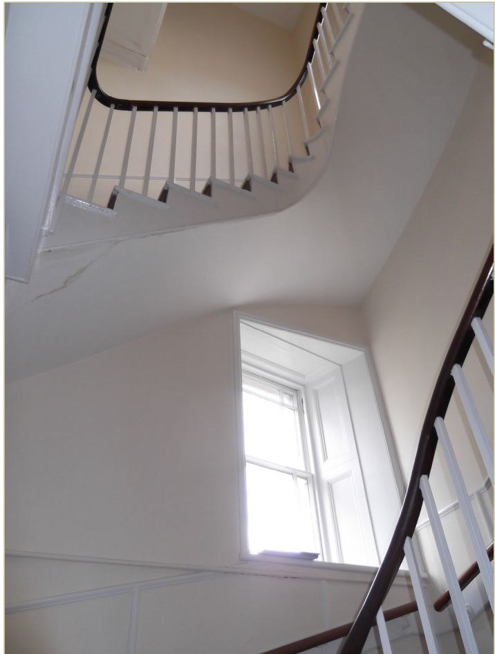
Figure 6. The staircase to 34 Beaumont Street
