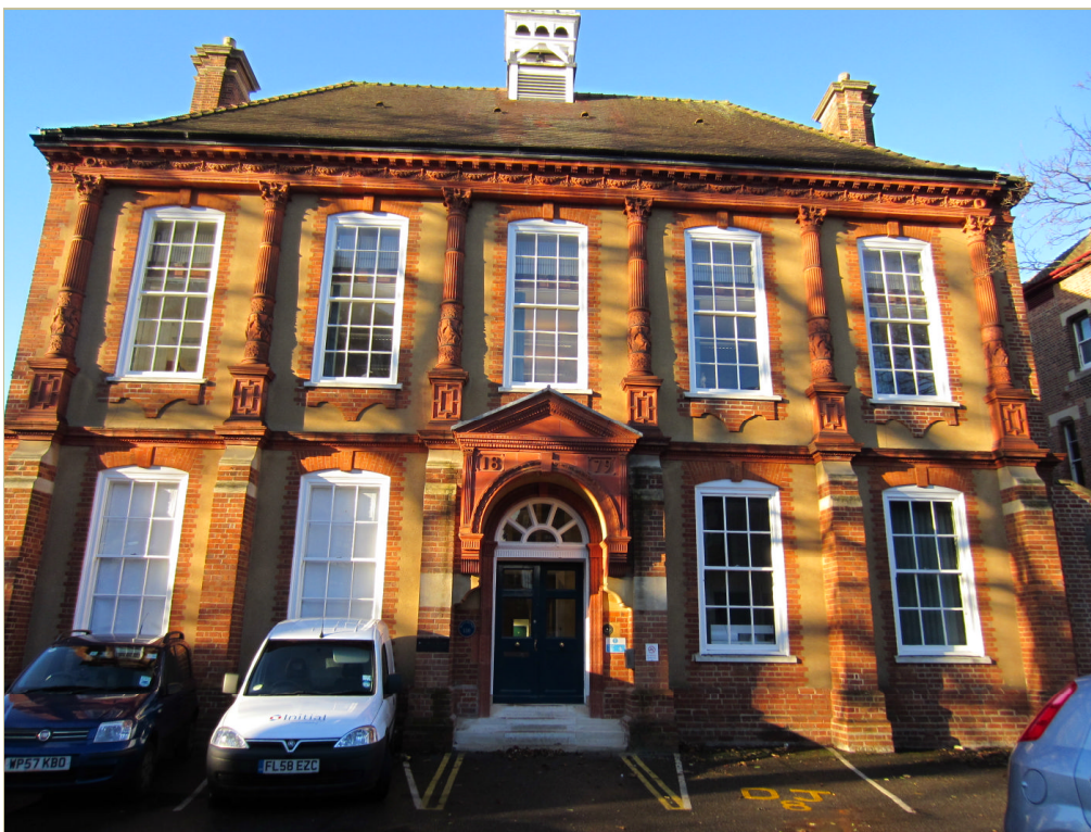
Figure 11. The primary façade of 21 Banbury Road
