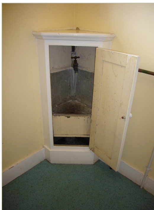
Figure 9. The caretaker's tap and basin on the first-floor landing of the rear staircase
