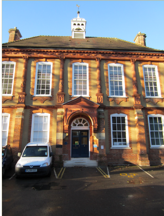
Figure 6. The eastern elevation
