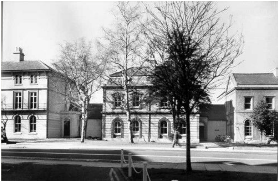
Figure 3. 9 to 15 Banbury Road in the late 1970s, showing newly-constructed connecting corridors.
