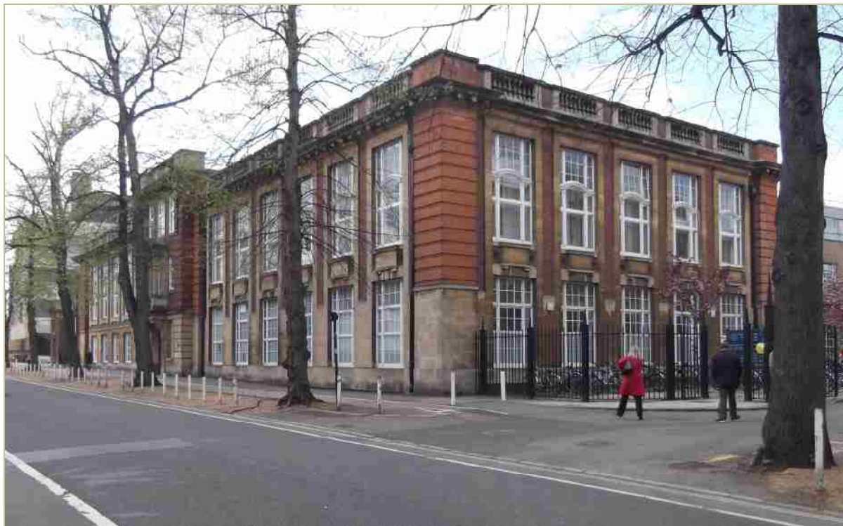
Figure 11. The Dyson Perrins Laboratory looking north-westwards from outside the Chemistry Research Laboratory
